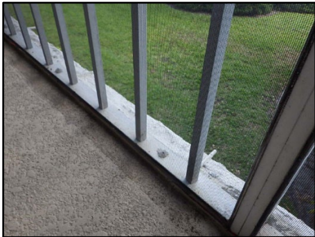
Balcony railing with lower edge screwed into concrete floor.
