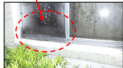
Roof runoff flows onto window.
