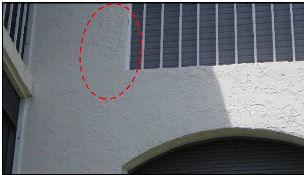
Crack in stucco on exterior of a balcony wall.
