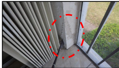
Cracked column on balcony.
