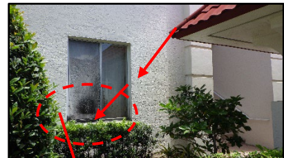
Roof runoff flows onto window.
