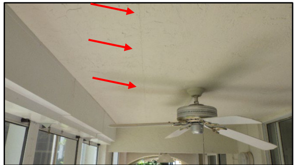
Hairline crack in ceiling along plank line. Not concerning
